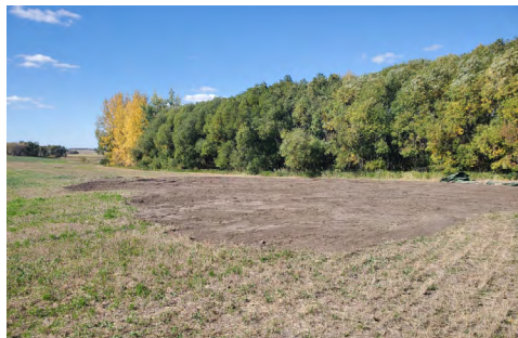
With backfill completed and the topsoil replaced, the land is ready to be returned to its pre-construction state.
