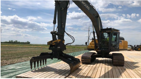
Decommissioning started in late May with rig matting to support cleaning of legacy Line 3.
