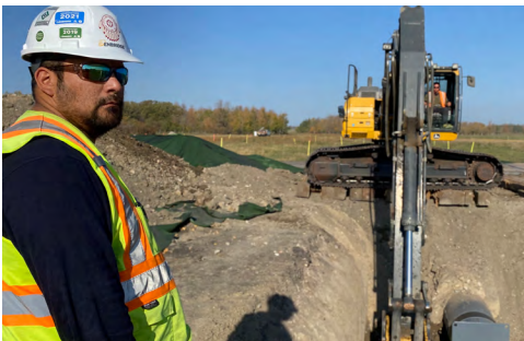
With the steel cap in place, Adam Cameron of Swan Lake First Nation looks on during backfilling.
