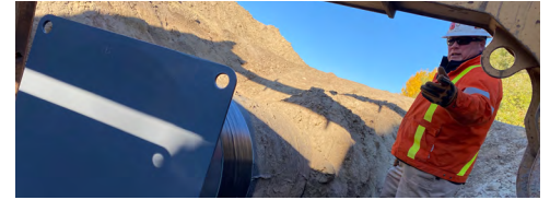
Inspector Sandy Armstrong shows a section of pipe following installation of a steel cap. After the pipe segment is cut, a cap is fabricated onto the ends of the pipe and coated with epoxy. This permanently seals the pipeline at that location and backfill can then be completed.
